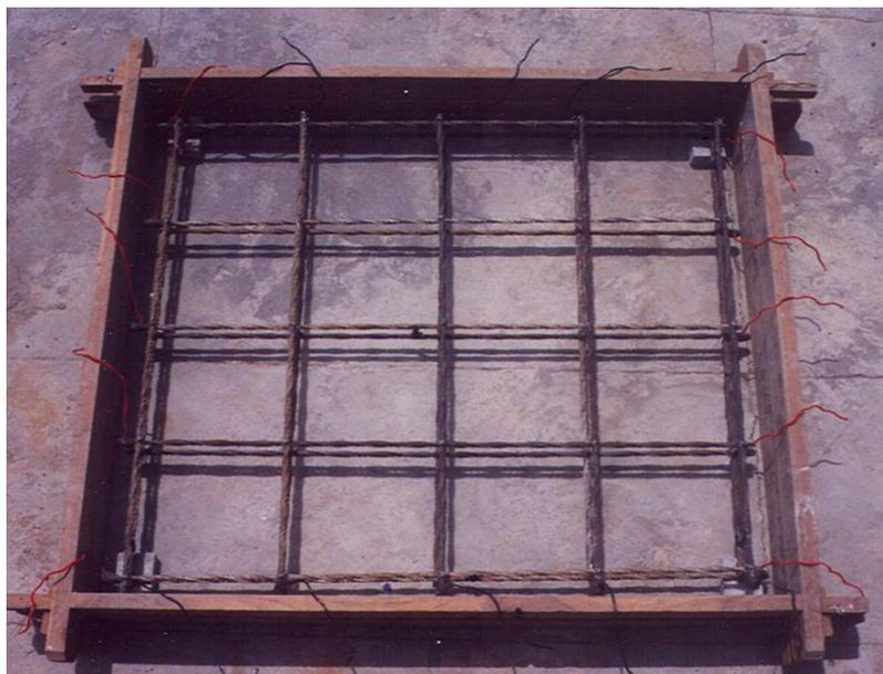
Rebar skeleton arrangement before placing concrete
