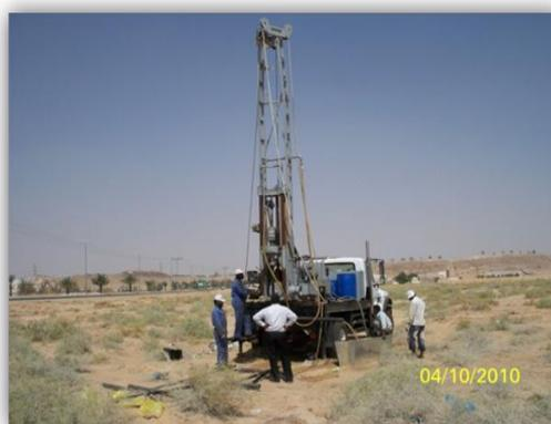
**Figure 4.** The conventional drilling using a truck mounted rig.
