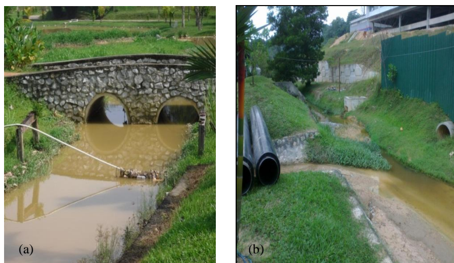
Figure 10. Monsoon drain (a) before construction and (b) during construction.
