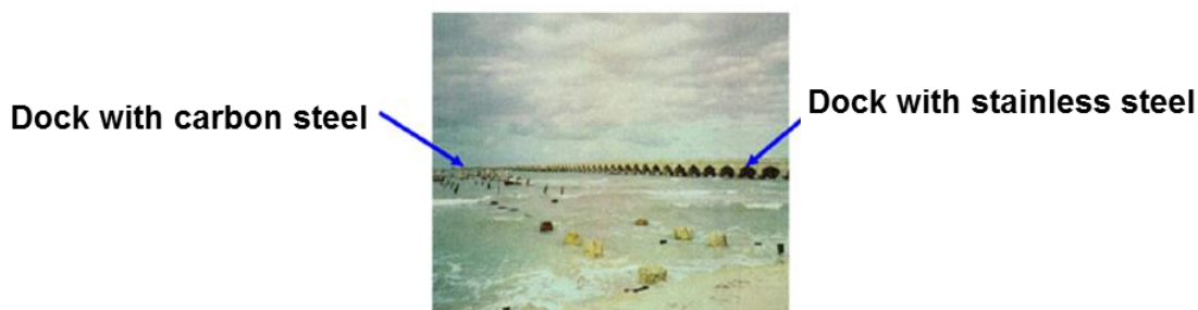
Figure 1. Stainless steel built dock on the right side, carbon dock on the left side of the image [12].
